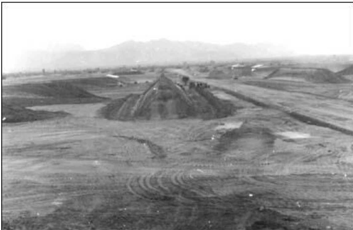
Phan Rang munitions storage area revetments, roads, and storage buildings, under construction. (1966)
